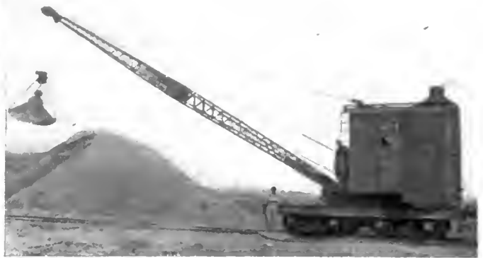
15 Ton Locomotive Crane.
